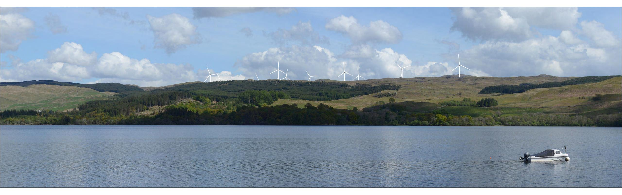
Photomontage showing current proposed layout. 13 turbines @ 180m to blade tip height.
