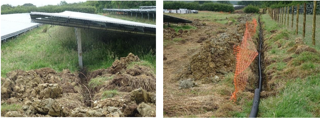
Photos 9 and 10: Cabling Channels During Cable Installation
