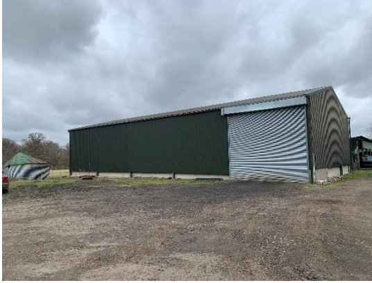
Photo 18 – 21: Farm Buildings, Little Cheveney Farm
