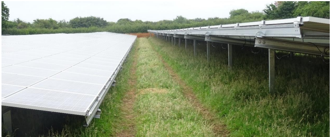
Photo 5: After Panels Bolted-on
