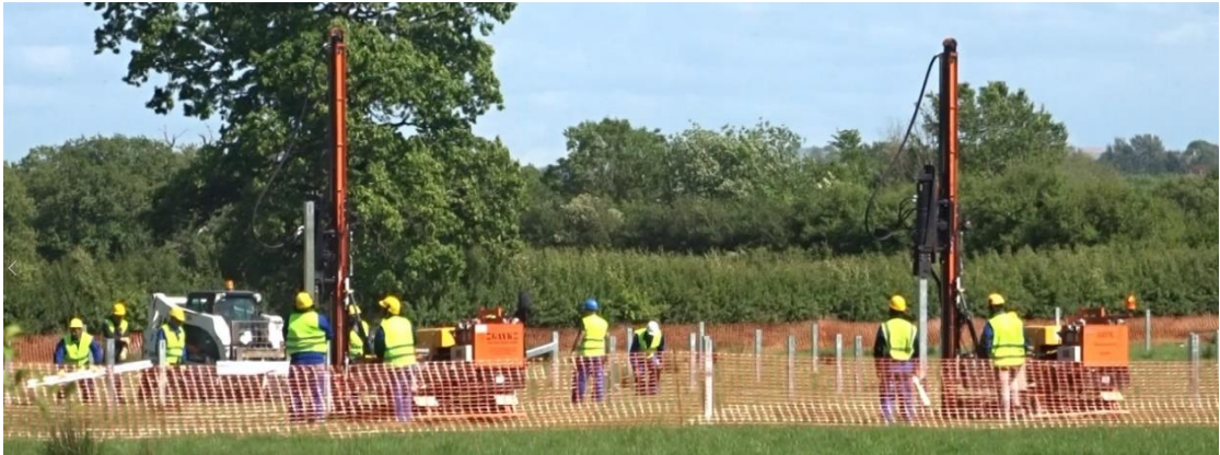
Photo 2: Legs Being Installed
