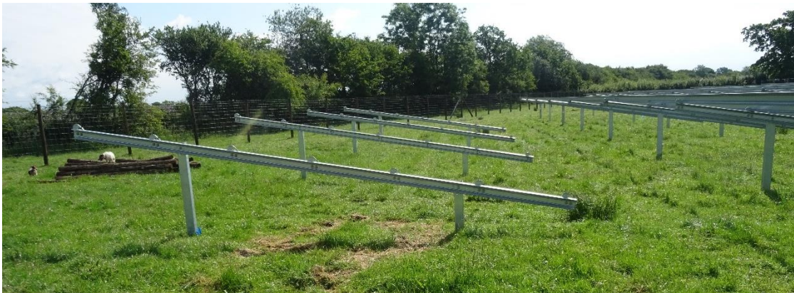
Photo 22: Legs Installed
