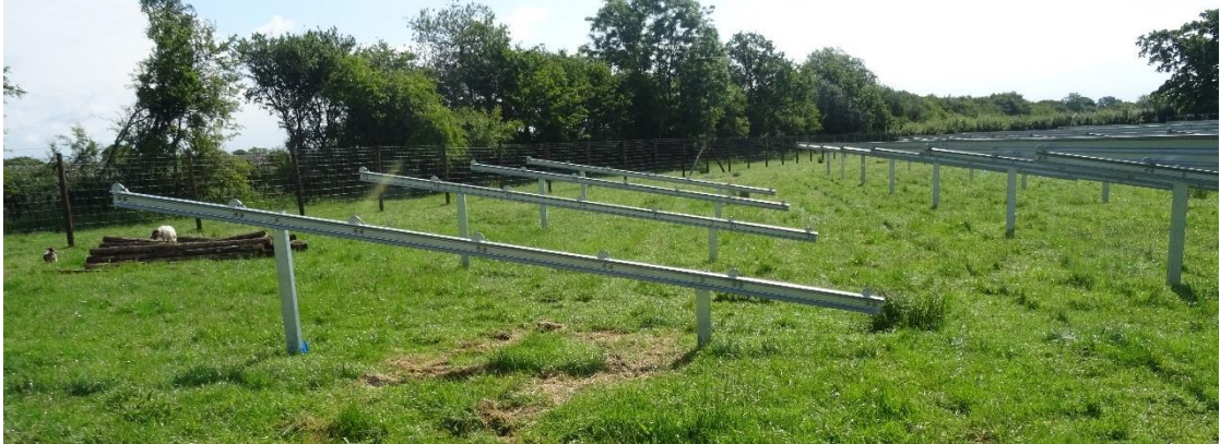
Photo 4: Legs Being Installed (this at Tiln Farm, Retford, in Janaury 2023)
