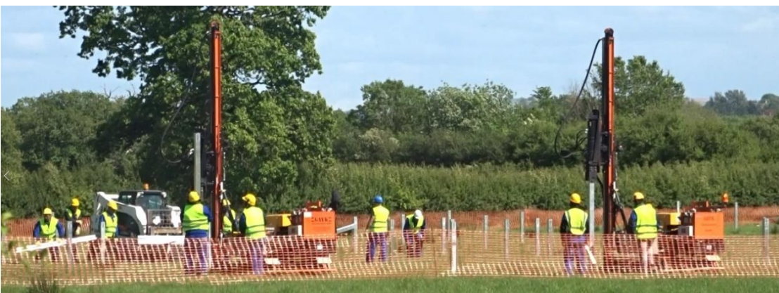
Photo 2: Legs Being Installed
