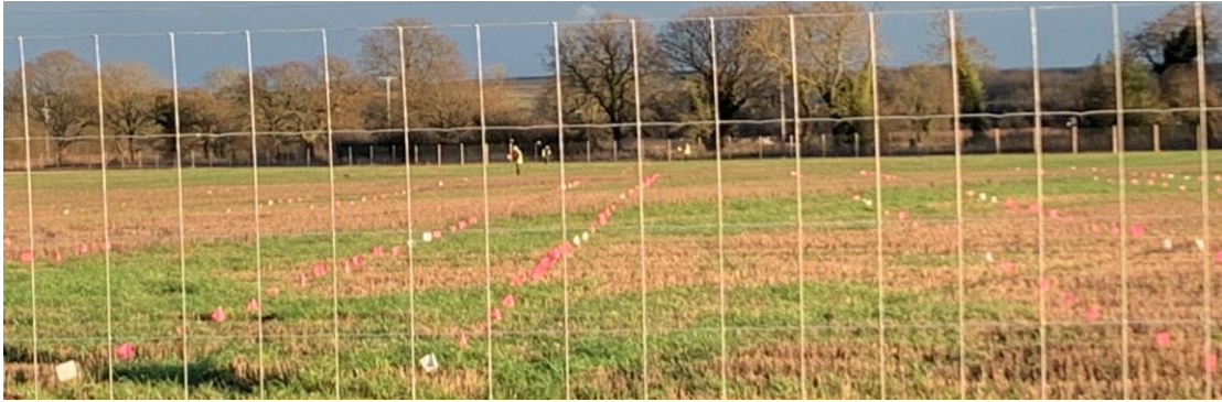
Photo 1: Marking Out in Progress
