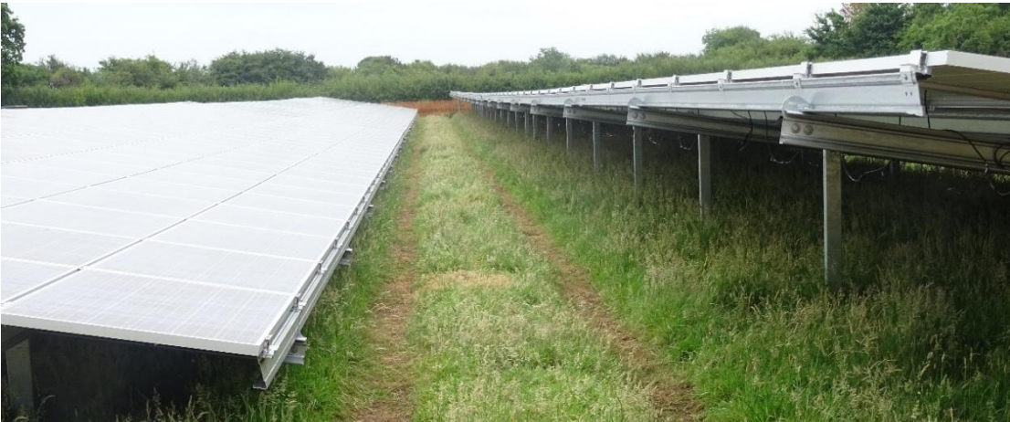
Photo 5: After Panels Bolted-on
