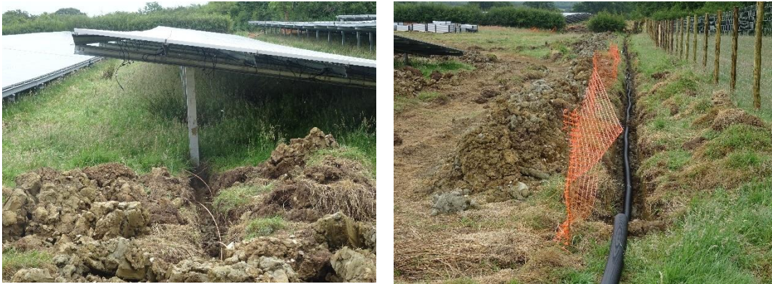
Photos 9 and 10: Cabling Channels During Cable Installation
