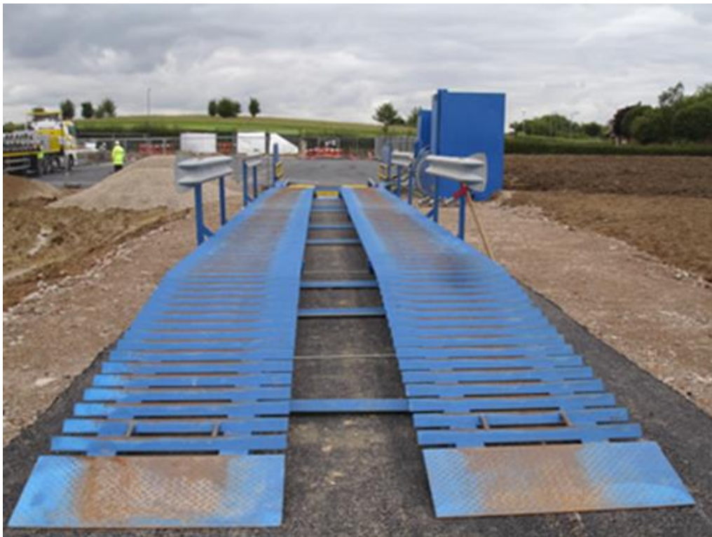
Plate 3.14: Vehicle wheel wash facility
