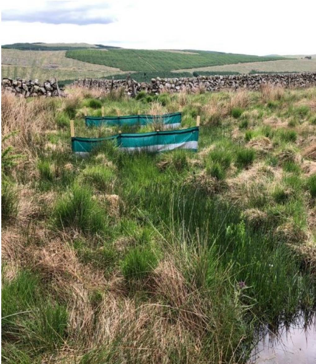
Plate 3.4: Typical silt fencing
