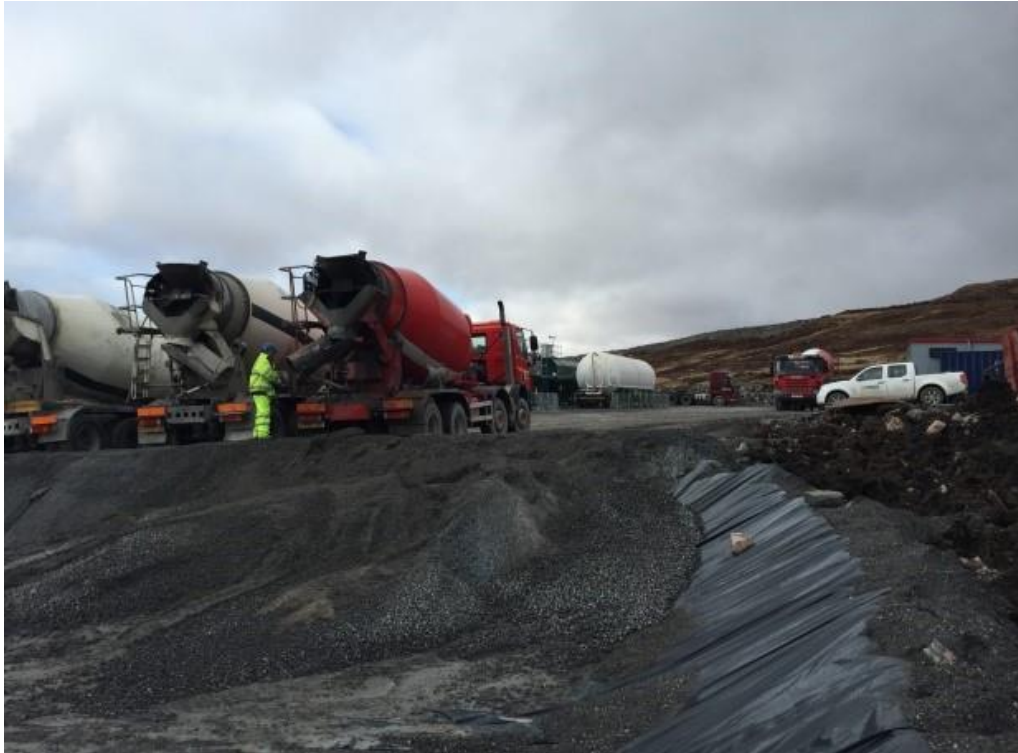
Plate 3.13: Concrete wash-out facility
