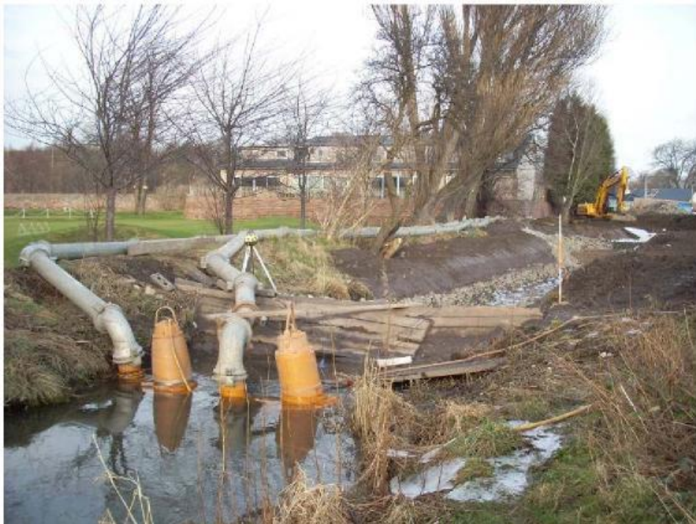
Plate 3.16: Watercourse Diversion (Full isolation – over pumping)
