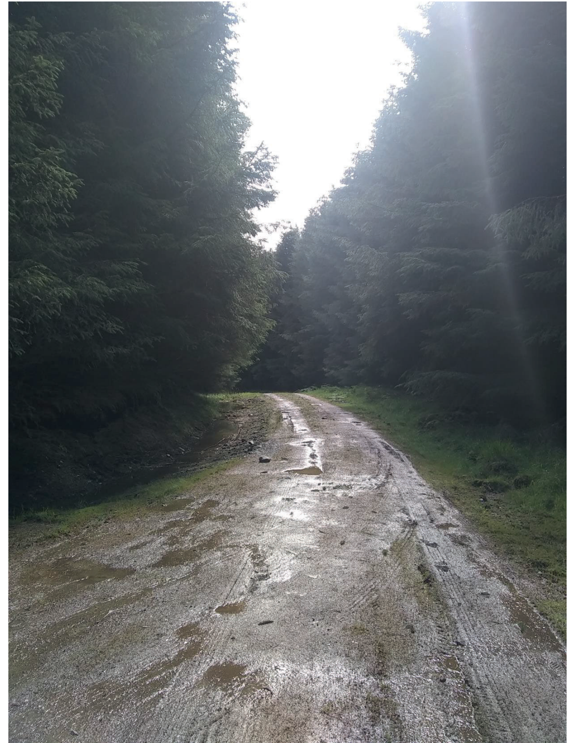
Plate 8: Existing forest track in western portion of the Site
