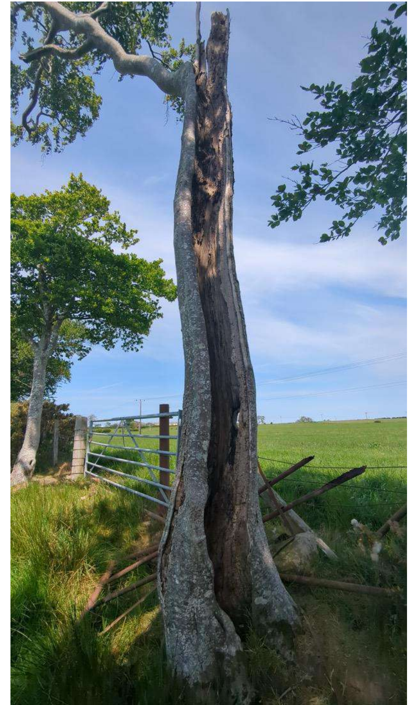
BS_050623 Coylton Substation Image No 06
