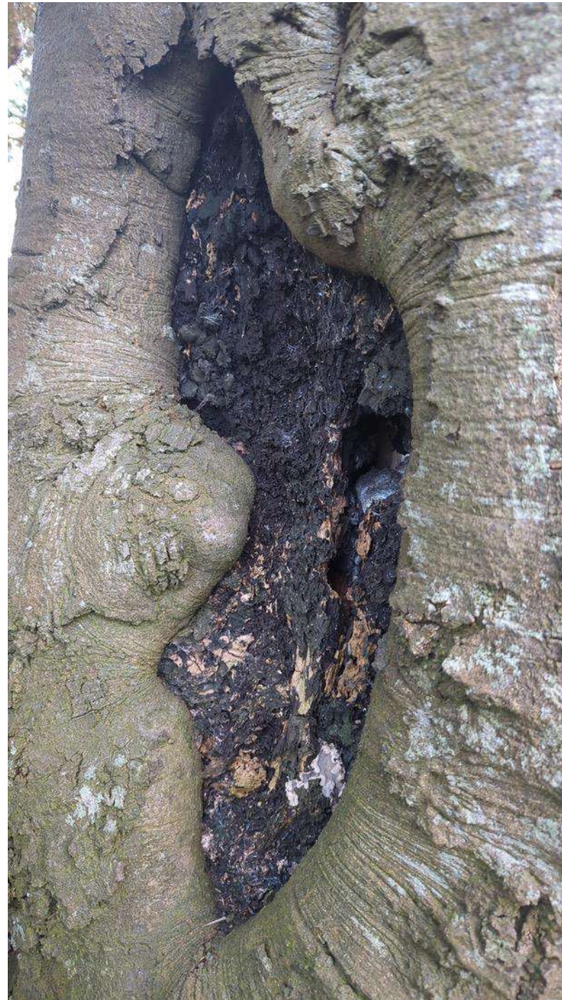
BS_050623 Coylton Substation Image No 05
