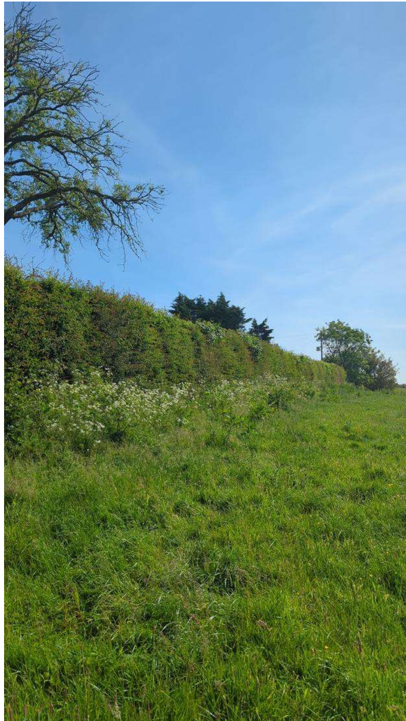
BS_050623 Coylton Substation Image No 07
