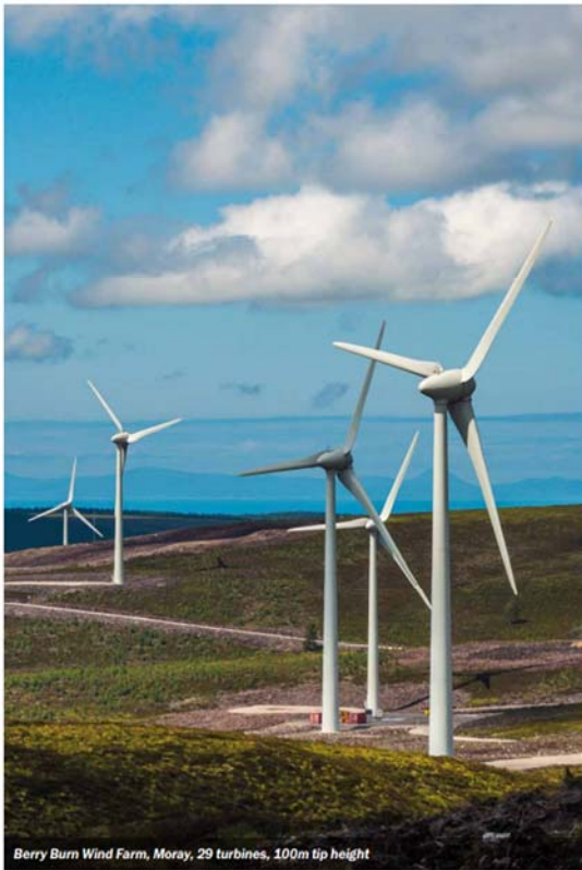
Berry Burn Wind Farm, Moray, 29 turbines, 100m tip height
