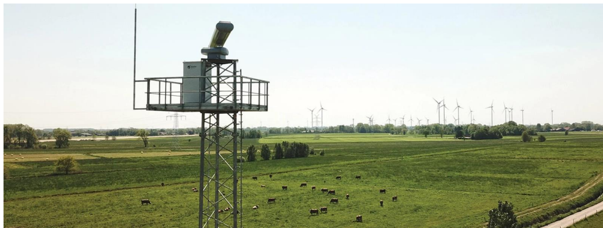
Figure 12 Terma 5002 Radar at a Wind Farm
