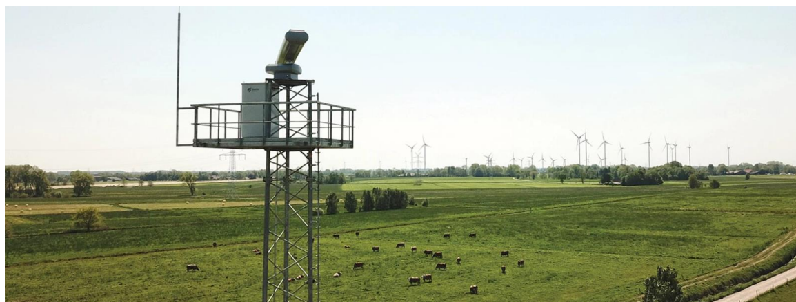
Figure 12 Terma 5002 Radar at a Wind Farm in Germany
