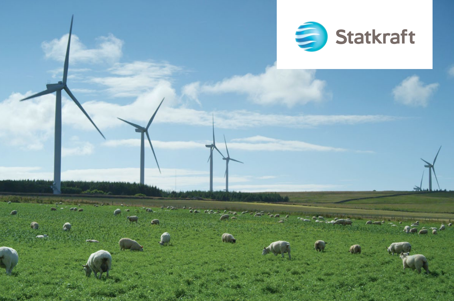
Baillie Wind Farm, Thurso, Scotland. 21 turbines. Installed capacity 52.5MW. Turbine tip height: 110m.
